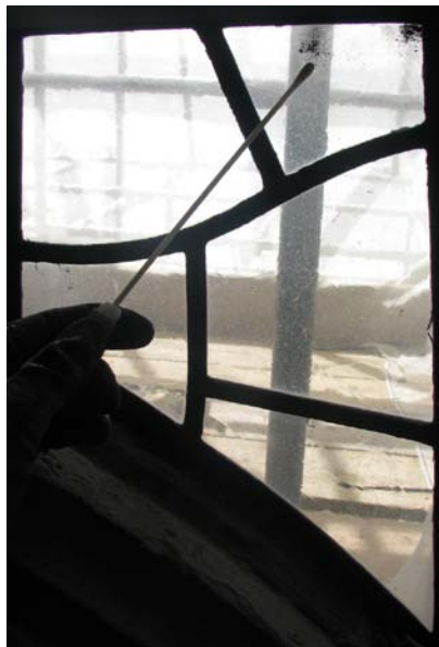
Taking swab from protective glazing panel
