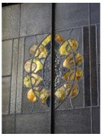
created by using: special rolled glass (fig.1), carved leading (fig.2), gilding form outside
